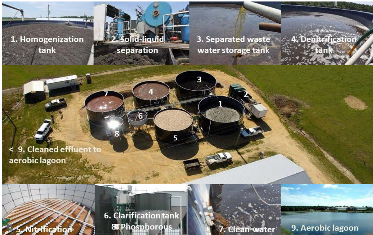
Exhibit 3-59: Nitrification Denitrification System
